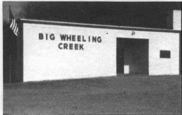
BIG WHEELING CREEK
